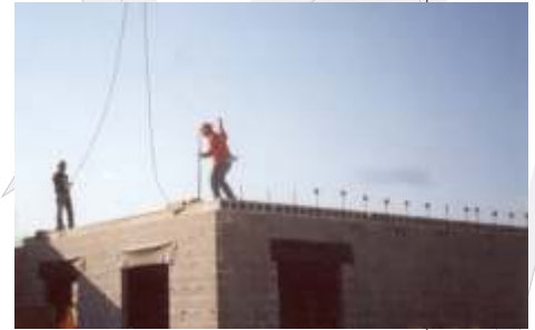
FEMA Tornado Proof Structure
