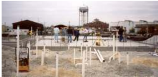
Basic Slab Prior to Reinforced Walls
